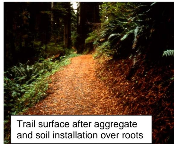
Trail surface after aggregate and soil installation over roots
