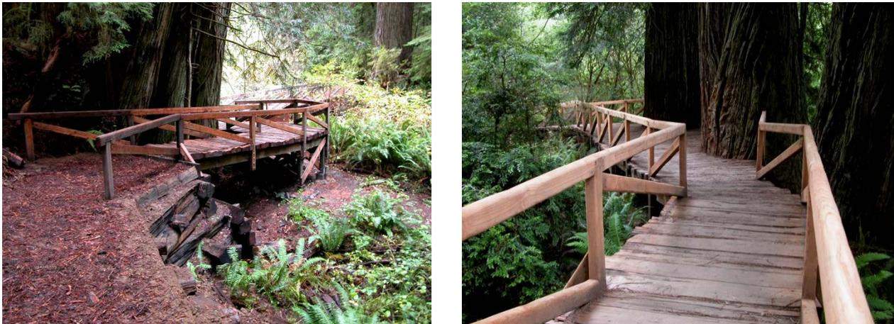
**Photo 8.15 - Use of Bridges to Maintain Linear Grade and Span Low Areas**
