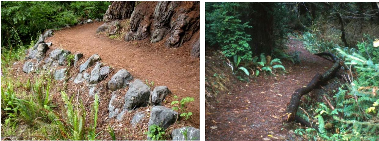
**Photo 8.22 - Using Native Materials to Provide Edge Protection**
