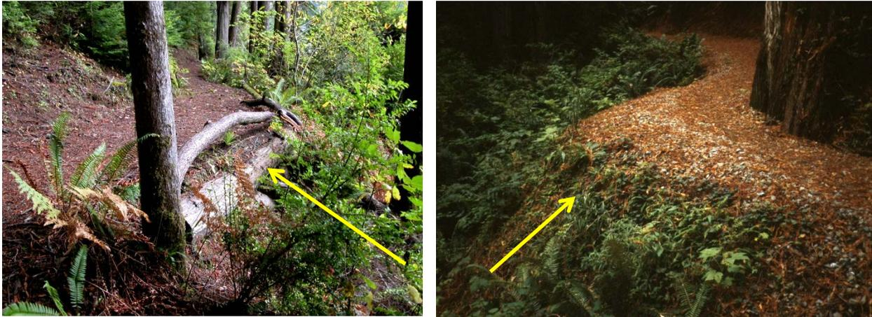
**Photo 8.14 - Use of Retaining Walls to Maintain Linear Grade and Protect Trees**
