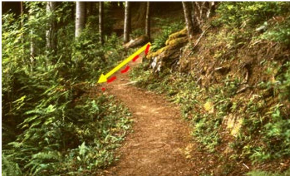
**Photo 8.13 - Combination of Linear Grade, Cross Slope, and Change of Direction**
